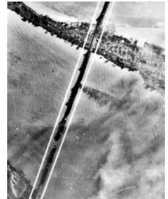
Post-strike RF-101 BDA = 1 rail and 2 highway spans down!
