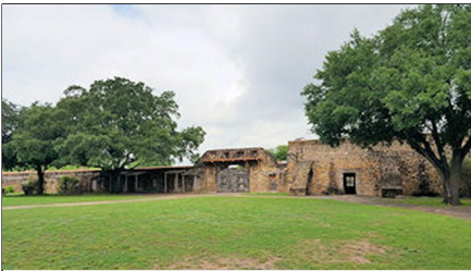
This is a close-up of various utilitarian buildings comprising part of the perimeter fortifications.
